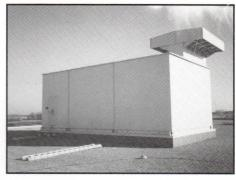
Air Conditioning Units • custom packaged air handling units continuing fans, heating and/or cooling coils, humidifiers and filters used for industrial heating and ventilating air supply, clean room air supply, and industrial process air supply requiring cooling and dehumidification.
